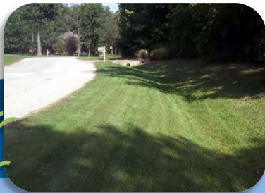
**Bioretention** is designed to filter stormwater runoff.
