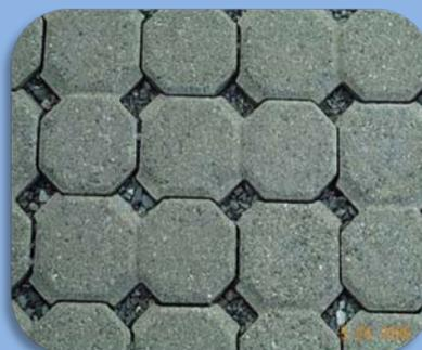
**Permeable pavers** allow the movement of stormwater through the surface that reduces runoff and filters pollutants from the water.
