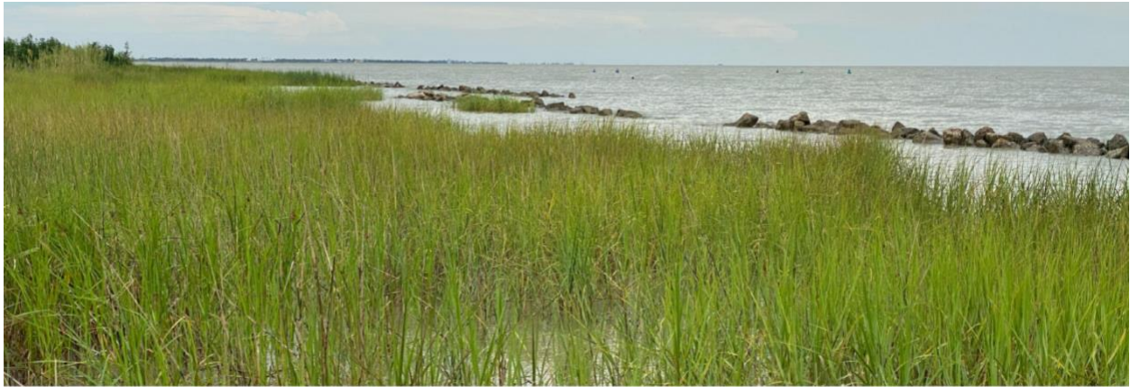
Figure 12. Image of a living shoreline protecting an existing marsh. Image from BCarbon.
